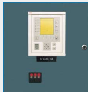
ABB type REF protection relay.
