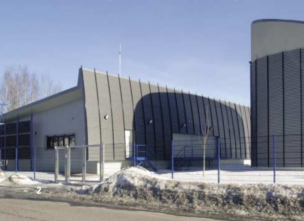
Innovac MMS power distribution, Kivenlahden, Espoo, Finland
